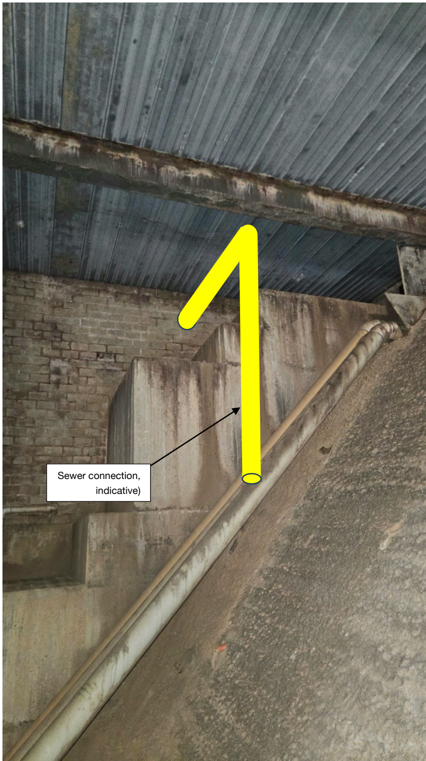
Photo 6 – View of void behind carpark where sewer will connect to existing (source: Kosciuszko Thredbo Pty Ltd).
